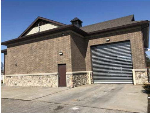
EXISTING BUILDING SOUTH ELEVATION
