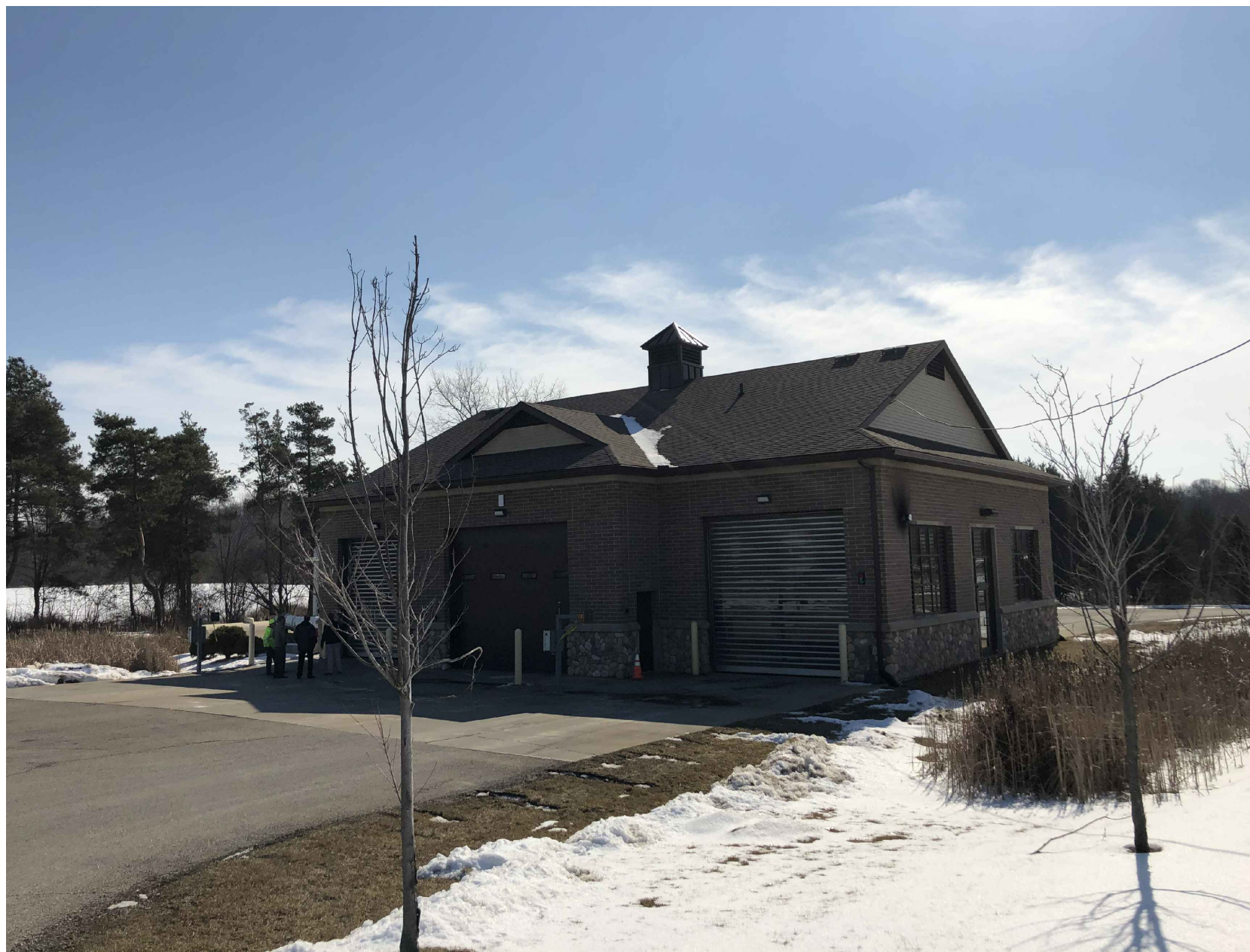
EXISTING BUILDING FROM NORTHWEST
