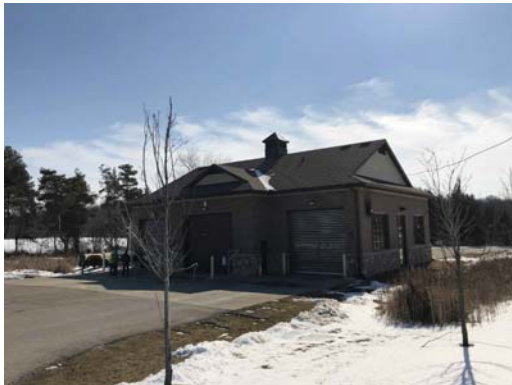
EXISTING BUILDING FROM NORTHWEST
