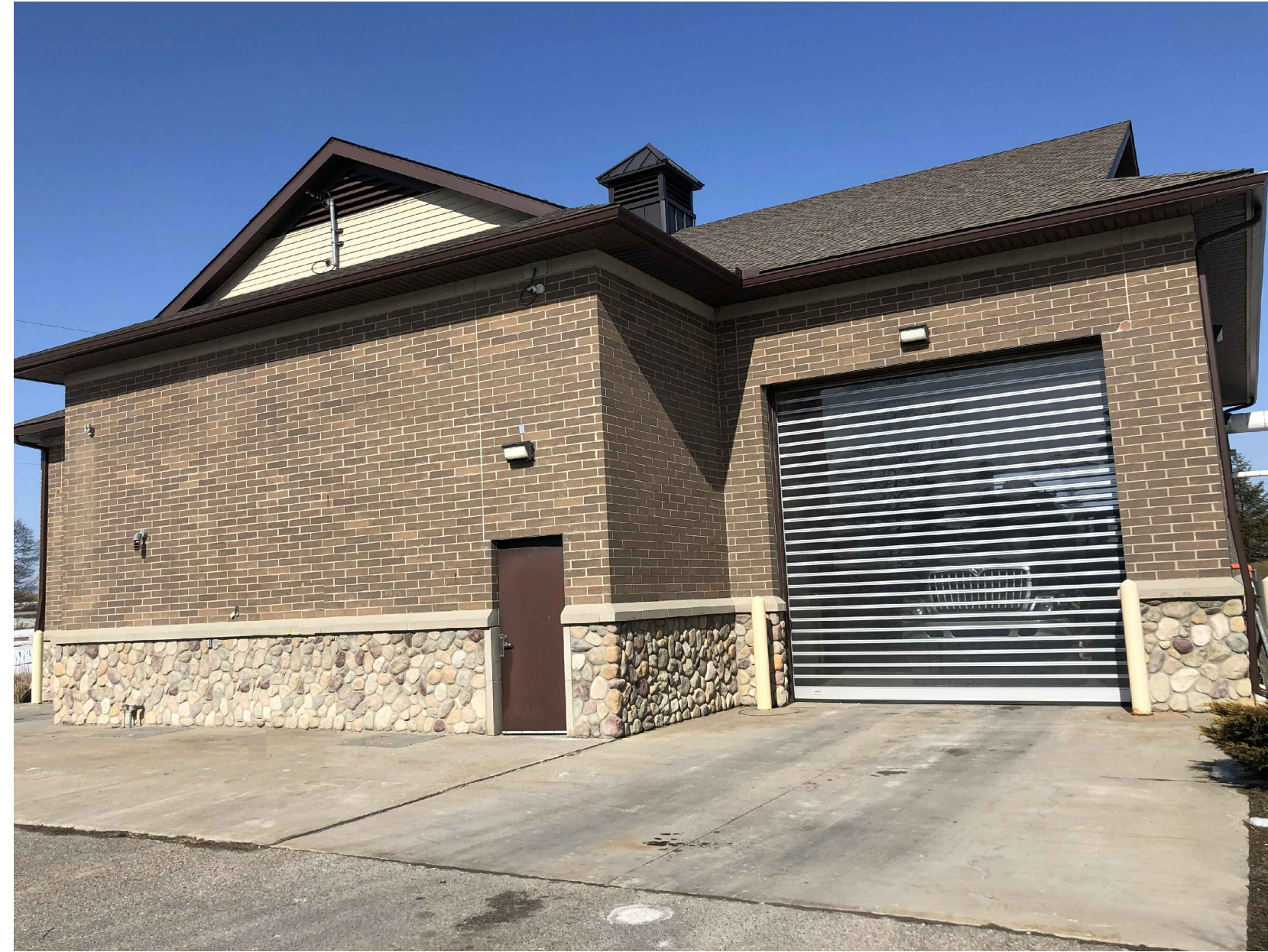
EXISTING BUILDING SOUTH ELEVATION
